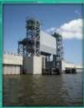
Intermediate Sections (15 Vertical Lift Gates)
